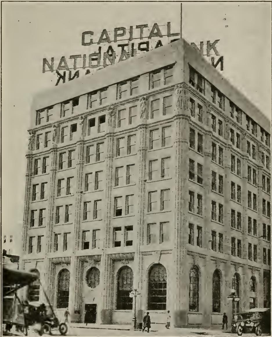
Capital National Bank Building, Sacramento, finished with architectural terra cotta from Steiger Terra Cotta & Pottery Works. Clay from pits in Amador and San Mateo counties.
